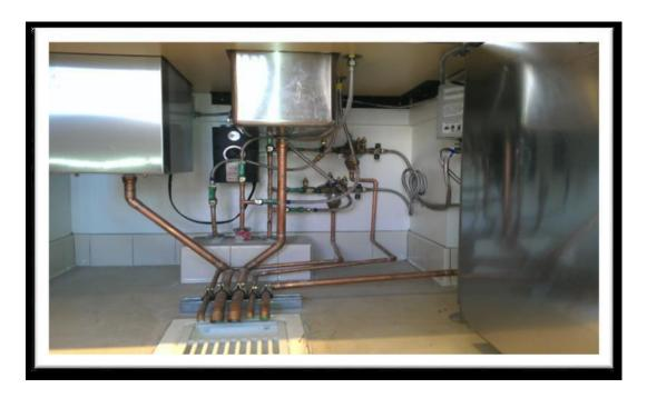
b) Warewashing sinks and warewashing machines shall drain to floor sinks unless the local building department requires a direct connection. When plumbed direct, connections to sewer must meet plumbing code requirements. See sample drawing below of Indirect Waste Drainage.
